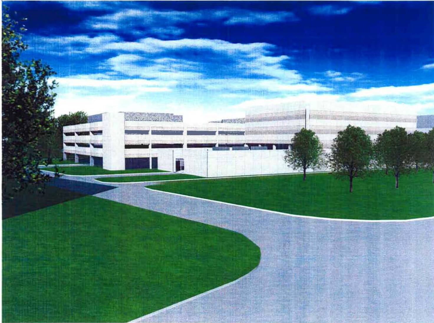
UTRP Utilities and Central Maintenance Facilities View From the Southeast
