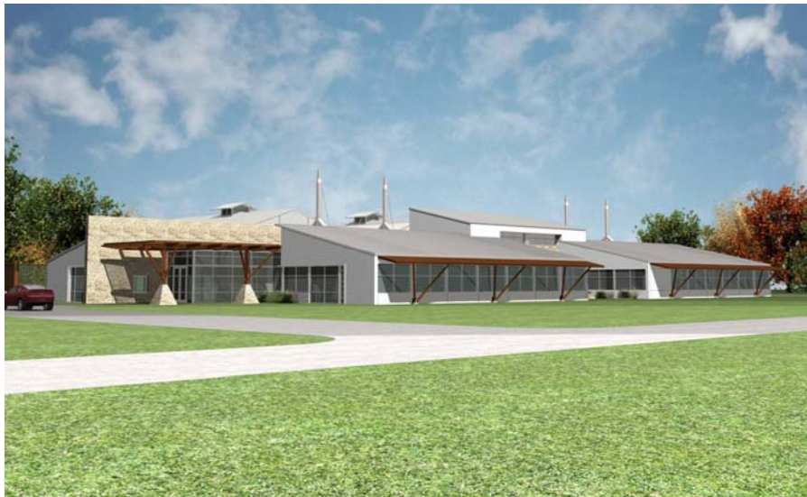
Bastrop Research and Education Building Northwest Perspective
