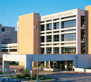
The Ambulatory Care Center at UT Health Science Center - Tyler
