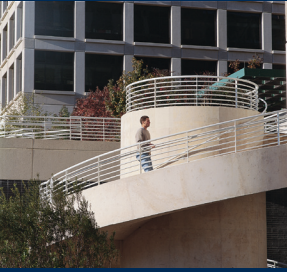
Stairwell leading to North Campus Plaza at UT Southwestern
